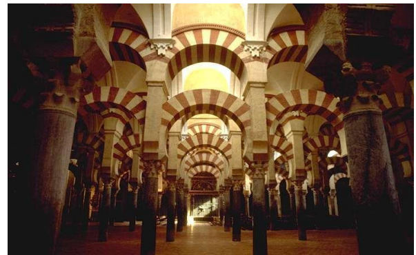
Figure 4. The funicular structure in the main room of the Cordoba Mosque building.
